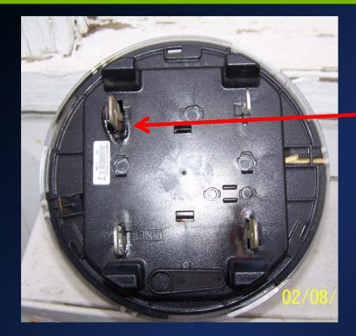
Heat from poor jaw connection flows through meter blade.
